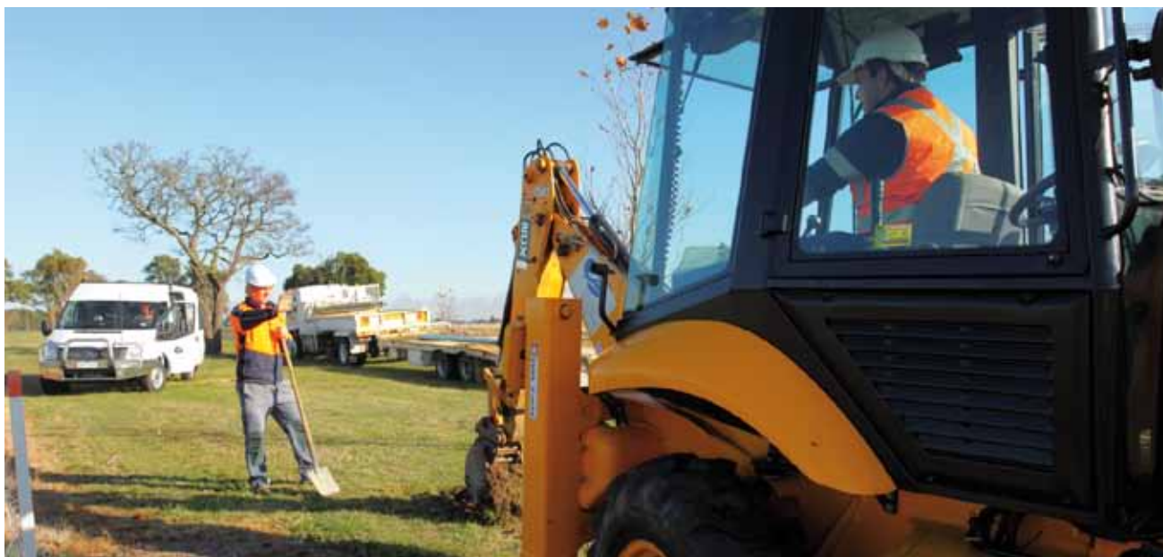
CHW staff commence water main repairs near Ballarat Airport.
